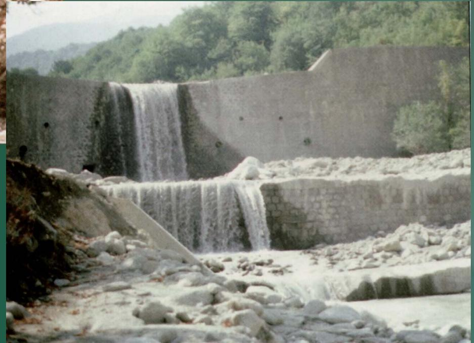
**Dam for erosion control in the
